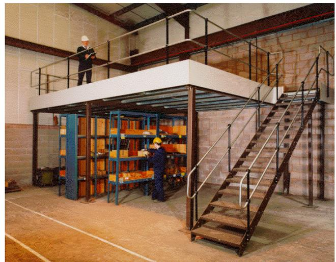
**Figure 1** A typical platform floor
